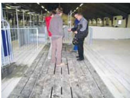
Rubber flooring from ErgoFloor (left), DUO slats from Sunds (right). Flooring is placed in the middle of the activity area where most fights for hierarchy arise.
